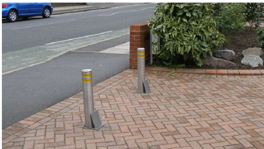
Lift up bollards, to be coated black
